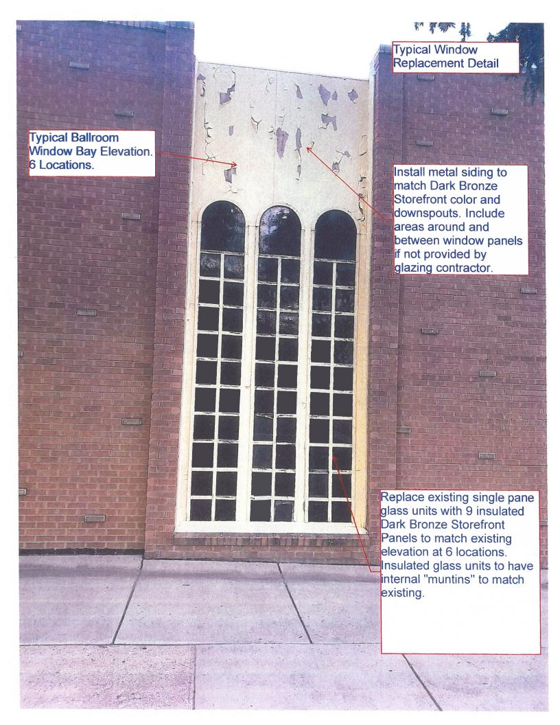
Typical Ballroom Window Bay Elevation. 6 Locations. Replace existing single pane glass units with 9 insulated Dark Bronze Storefront Panels to match existing elevation at 6 locations. Insulated glass units to have internal "muntins" to match existing.
